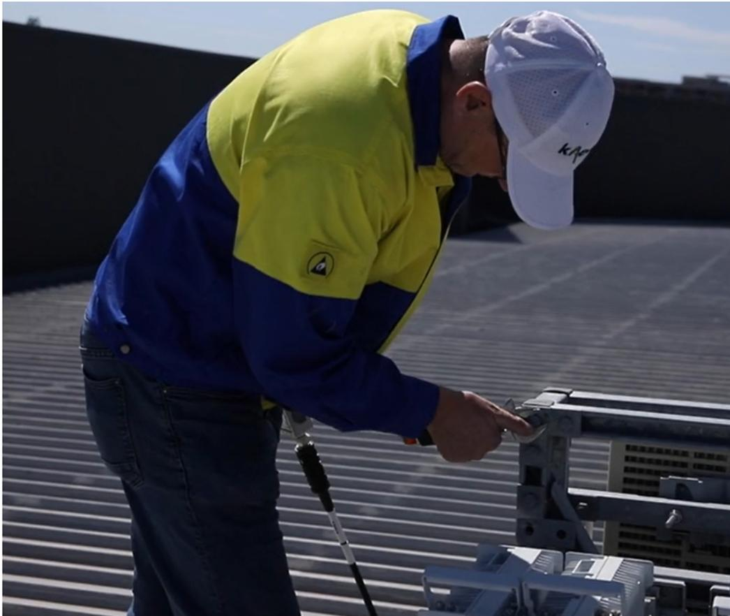
Essentially any metal-to-metal contact should be inspected to ensure no intermittent connection.
